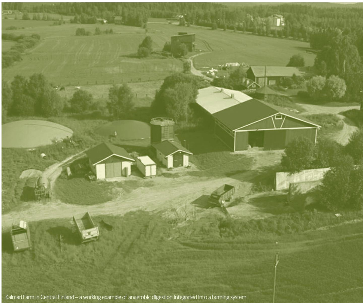
Kalmari Farm in Central Finland – a working example of anaerobic digestion integrated into a farming system
